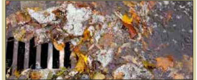
The public is encouraged to remove leaves and other debris from storm drains to prevent localized flooding.
