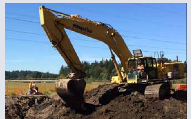
Excavator at work on the Kinsman Road Extension project.
