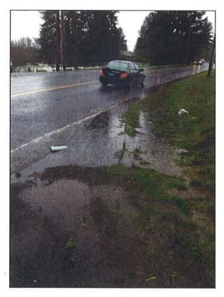
Photo C2. At top of photo is the original Washington County culvert outlet under Boones Ferry Road discharging to the west (December 2012). This is an old concrete pipe. The pipe at the lower-left portion of the photo is the plastic pipe draining onto the Lucini property.
