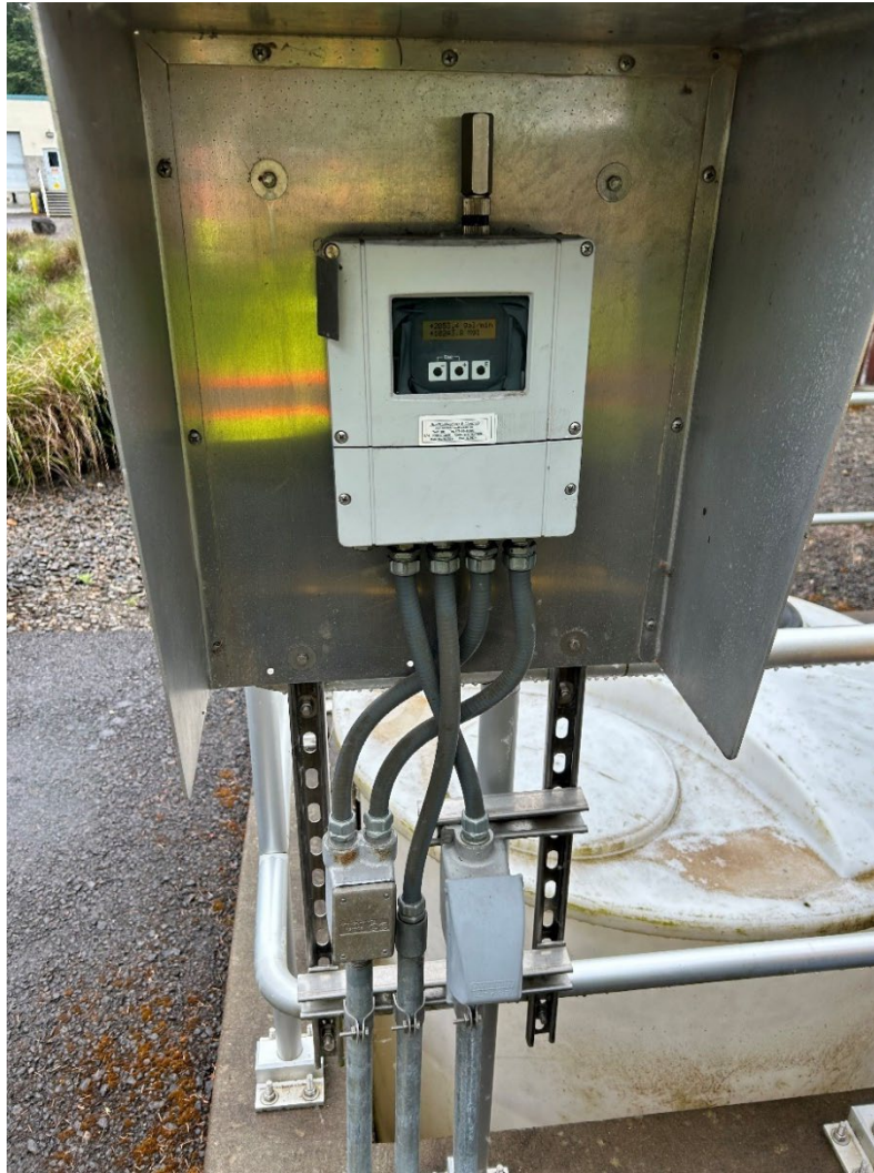
Figure 3-7. Flow meter display
