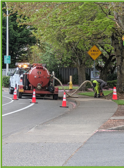
Operating the Ditch Witch
