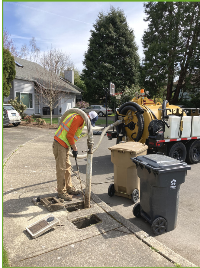
Sam cleaning out meter boxes
