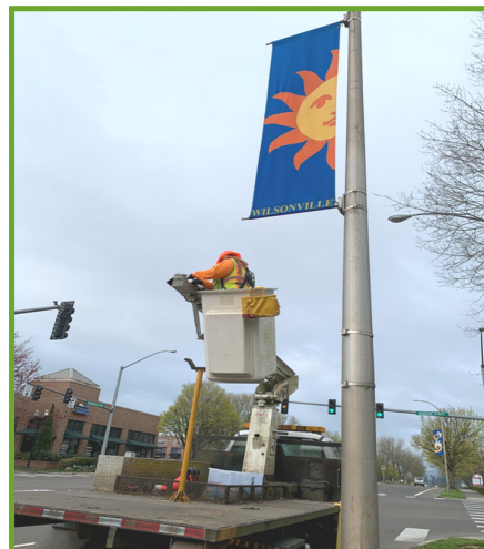
Coming down in the bucket lift
