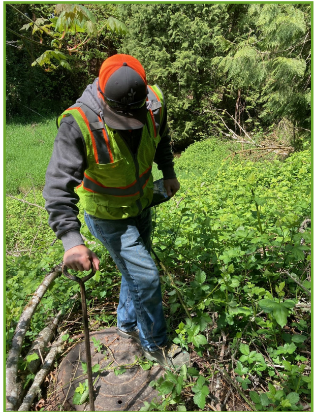
Randy lifting a manhole lid
