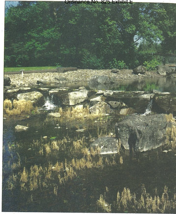
The 16-year-old Willamette River Water Plant has the ability to ozonate inorganic contaminants.
